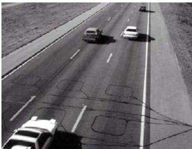
Fig. 1: Inductive loop detectors
